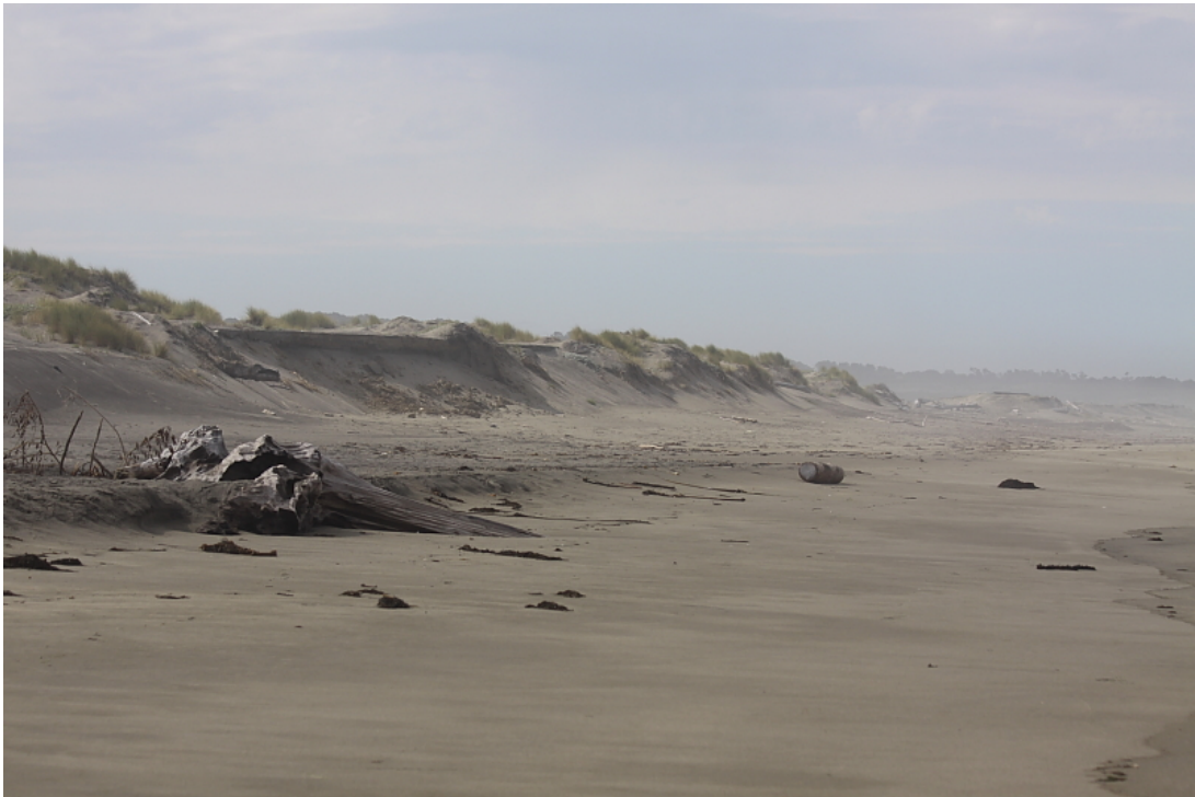
Remnant section of old Haul Road and eroded asphalt. August 2012.
