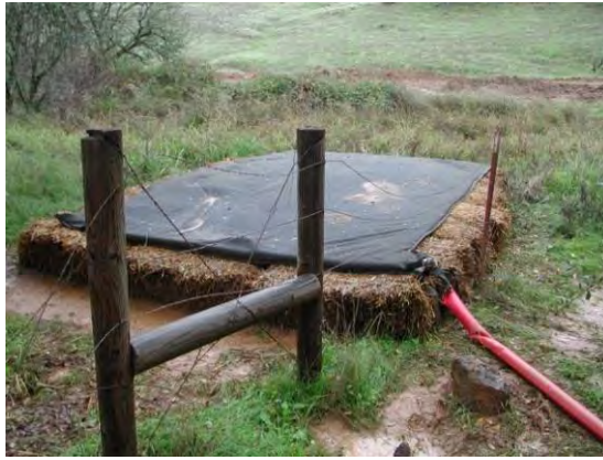
Figure 3.HYDRO.a-01: Typical Setup of Sediment Capture Bag
