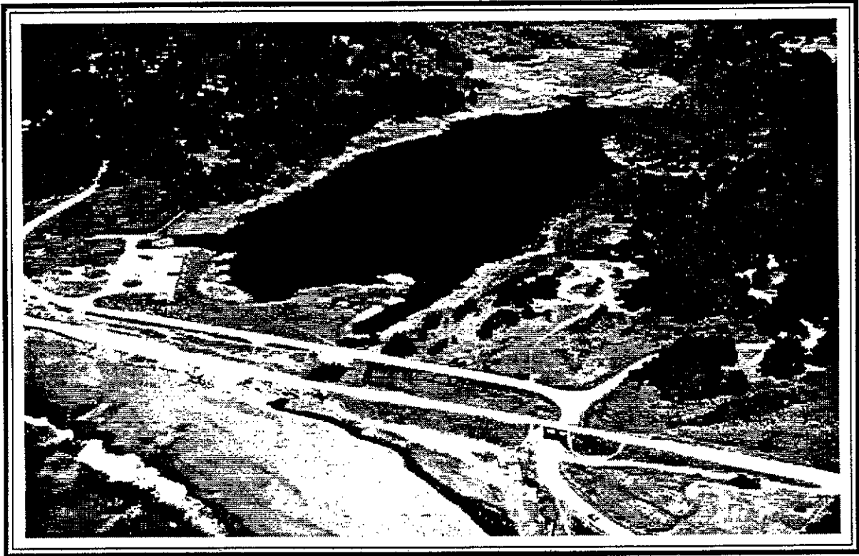
Lake Cleone and its surroundings from the air. Clockwise from the lower lefthand corner are MacKerricher Beach, the haul road berm, the park road, the Lake Cleone parking lot, the slope north of the lake, the freshwater marsh east of the lake, Surfwood Campground, and the park road underpass beneath the haul road berm providing access to Laguna Point.
